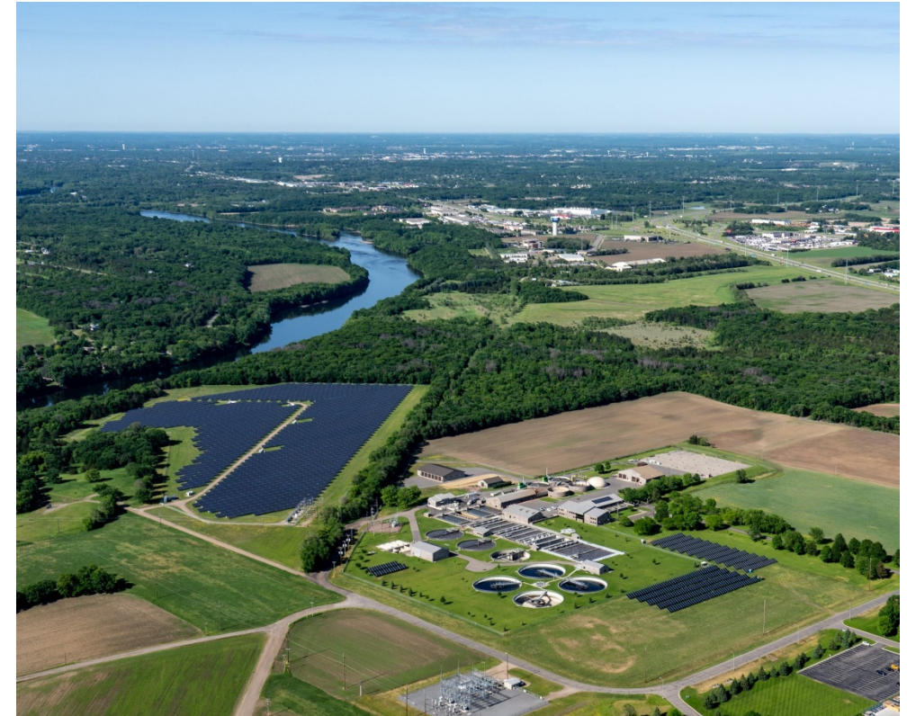
St. Cloud wastewater treatment facility
